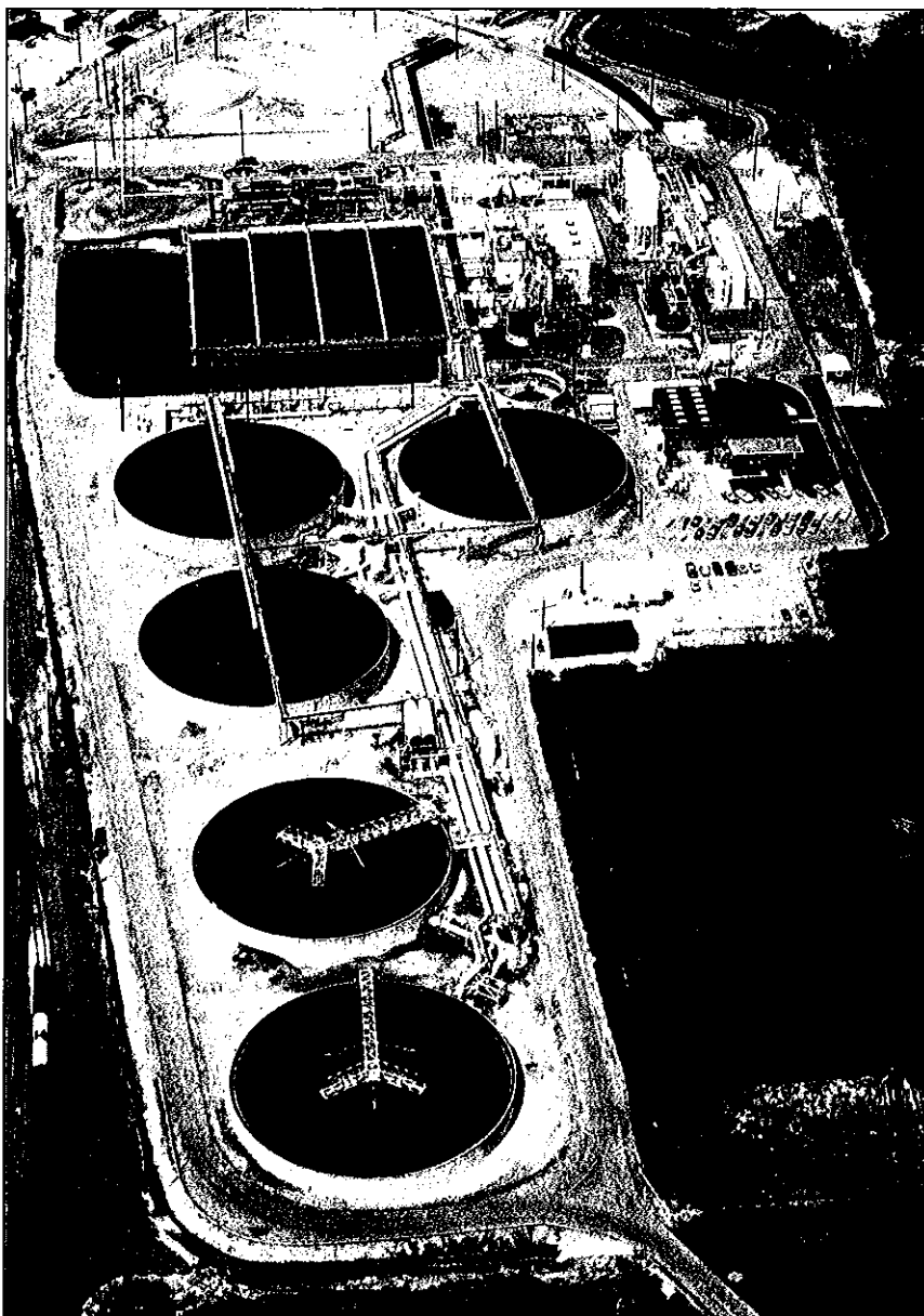
Figure 1. Aerial view of DuPont's chamber works treatment plant.
