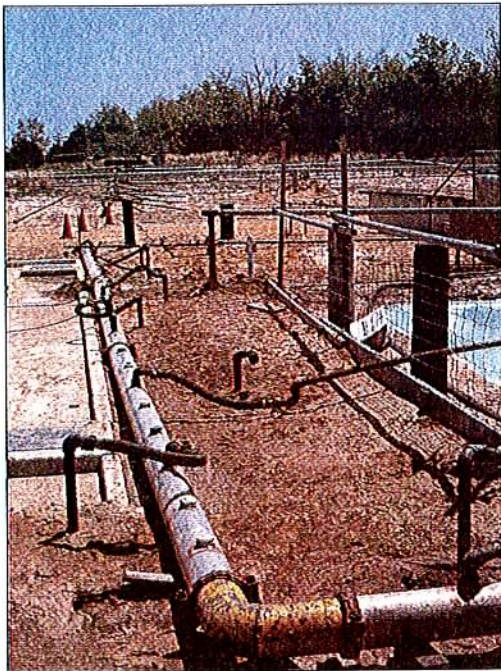
Electrolytic respirometry studies verified that in situ biological treatment was a viable option for remediating ethylene glycol-contaminated groundwater.
